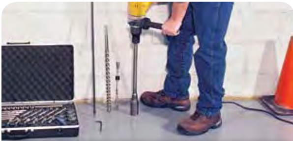
1. Create a 1/8" recess hole with the core bit so that the tamper-resistant cap will fit flush with the floor surface when installed.
