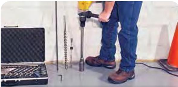
1. Create a 1/8" recess hole with the core bit so that the tamper-resistant cap will fit flush with the floor surface when installed.
