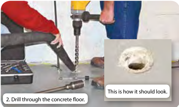
1. Create a 1/8" recess hole with the core bit so that the tamper-resistant cap will fit flush with the floor surface when installed.
