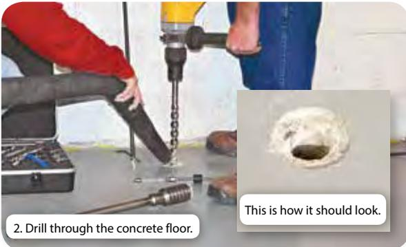
2. Drill through the concrete floor.
