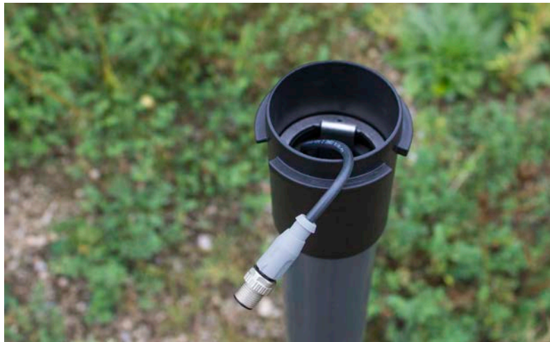
Figure 6-6 Lower the Assembly into the Well
