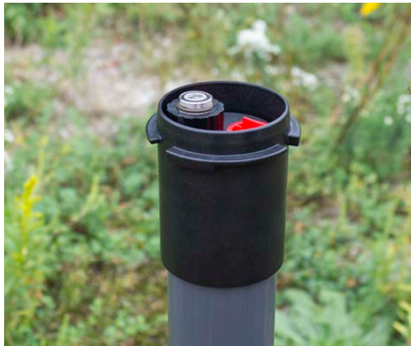
Remove Existing Levellogger Installation
