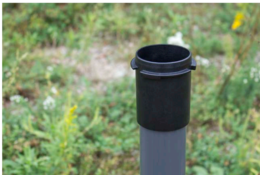
Figure 6-3 Install the Well Cap Base
